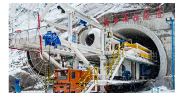
Entrance of Duoxiongla Tunnel of Paizhen-Motuo Highway in Tibet
