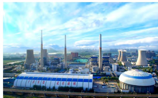
Huangtai Power Plant in Shandong province
