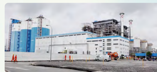
Tembusu Power Plant in Singapore
