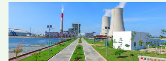
Green Landscape of Sahiwal Coal-fired Power Plant
