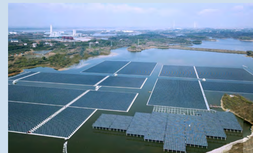
Sanhui Lake Water-Surface Photovoltaic Power Station in Hunan
