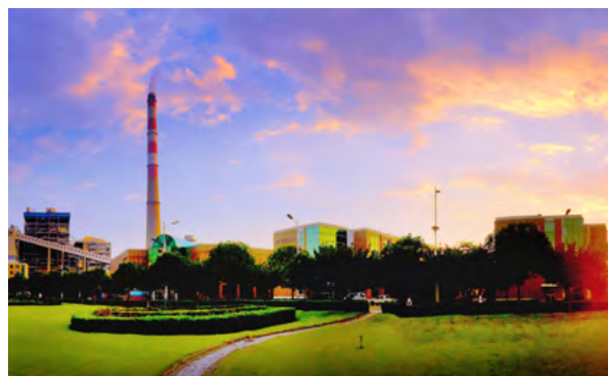
Hanfeng Power Plant in Hebei province
