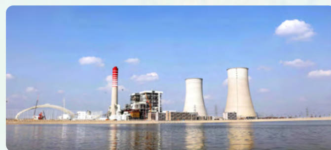
Pakistan Sahiwal Coal-fired Power Plant
