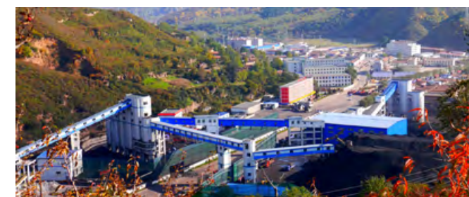
Industrial Site of Xinyao Coal Mine
