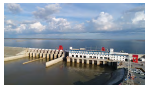
Lower Sesan River II Hydropower Station
