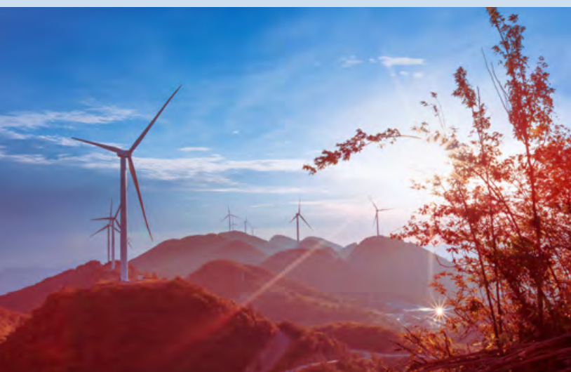
Jinfeng Mountain Wind Farm in Chongqing
