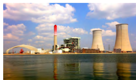
Pakistan Sahiwal Coal-fired Power Plant
