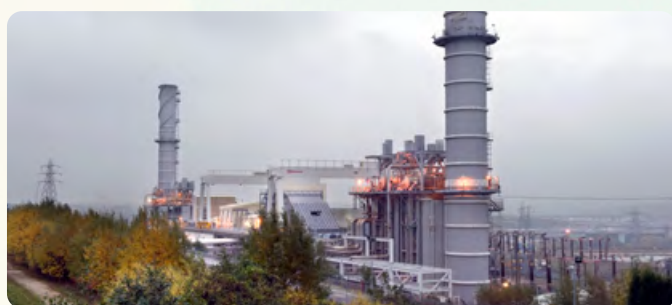
Rocksavage Power Plant in the UK
