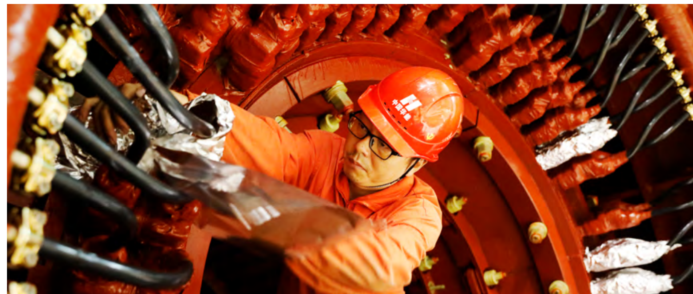
Personnel of Zhejiang Branch carries out condition-based maintenance to ensure safety
