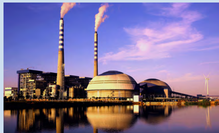
Hainan Dongfang Power Plant
